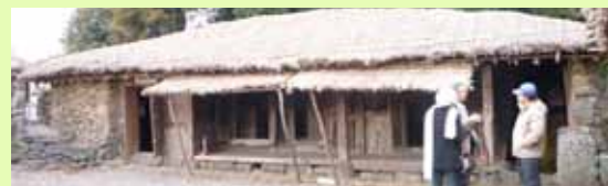
The Jeju state government gave incentives and support for traditional architecture preservation and restoration in Seoungueup Folk Village
