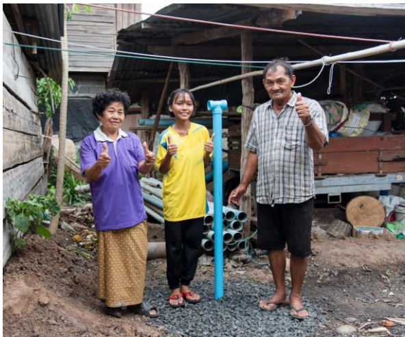
Water supply improvement
