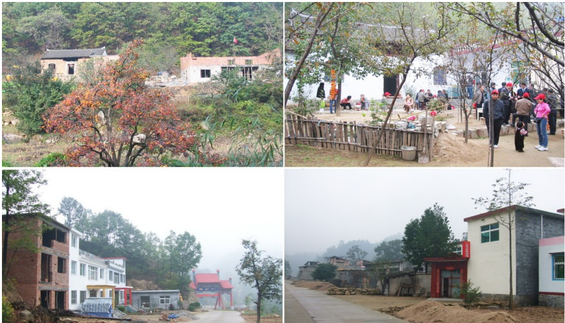
Top: A new house being built as a family hotel (left). Family Hotel 2 was hosting a group of tourists (right). Bottom: The nearly completed construction of a new family hotel (left) and Family Hotel 5 (right).
