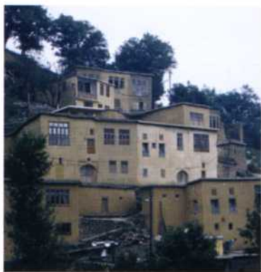
Houses in the village of Masouleh in Iran's Gilan Province are built on top of each other up a steep hillside.
