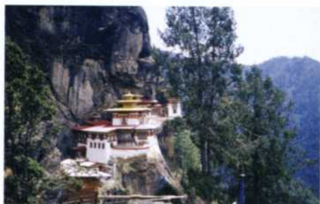
Clinging dramatically to the side of a high cliff, the Taktsang Monastery is one of the most important religious sites in Bhutan. © David Tresilian
